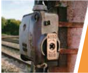
A signal post replacement switch
